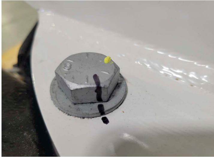
Figure 3-7. Marking Bolt Heads Prior to Torque Check
